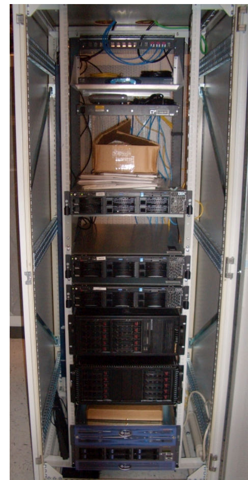
ASF Rack, UnitedLayer Co-Location
